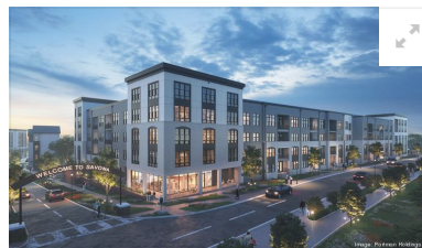
Portman Residential's renderings for phase one of its Savona Residences project, part of the Savona Mill redevelopment.
